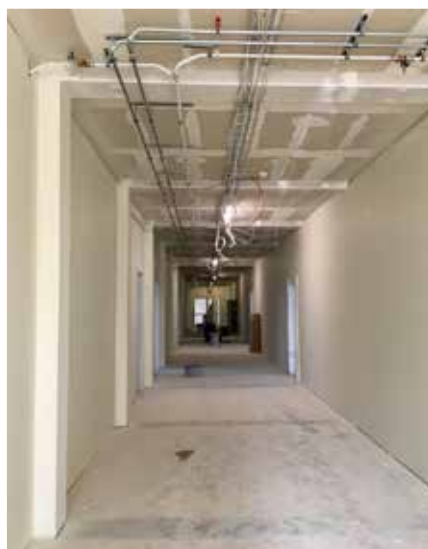
Modulbau Phase 2 innen
